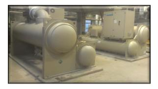
The upgrade to the centrifugal chiller plant included the installation of two Daikin WME700 chillers (above) with
